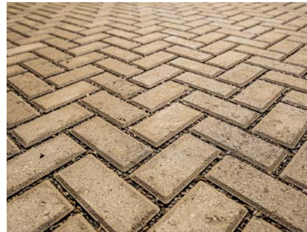
Pavers with Crushed Gravel
