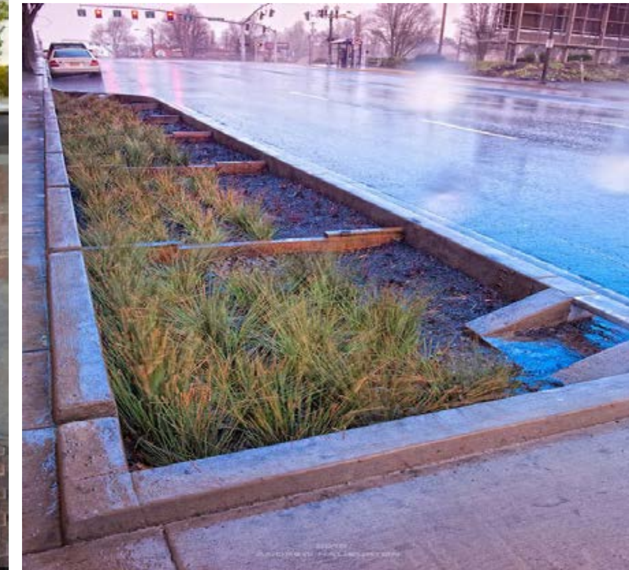
Concrete Check Dam
